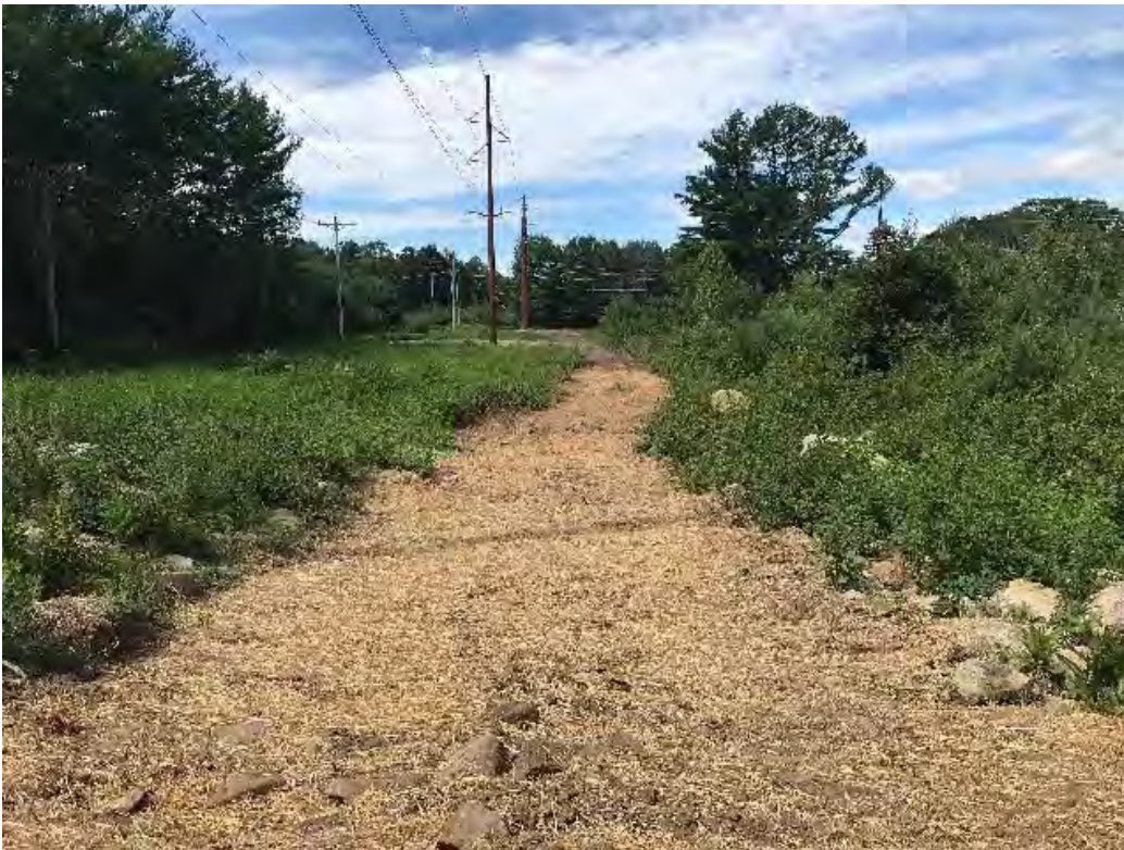
Fig 6: Access road from Strs. 50 to 49 seeded and mulched. Viewing southwest. (08-03-20).
