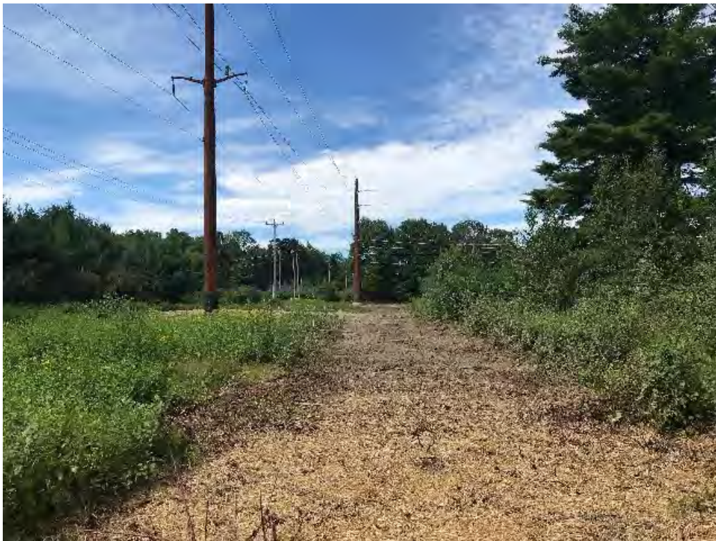
Fig 4: Access road across wetland DW54. Timber mats removed and wetland seeded. View southwest. (08-03-20).
