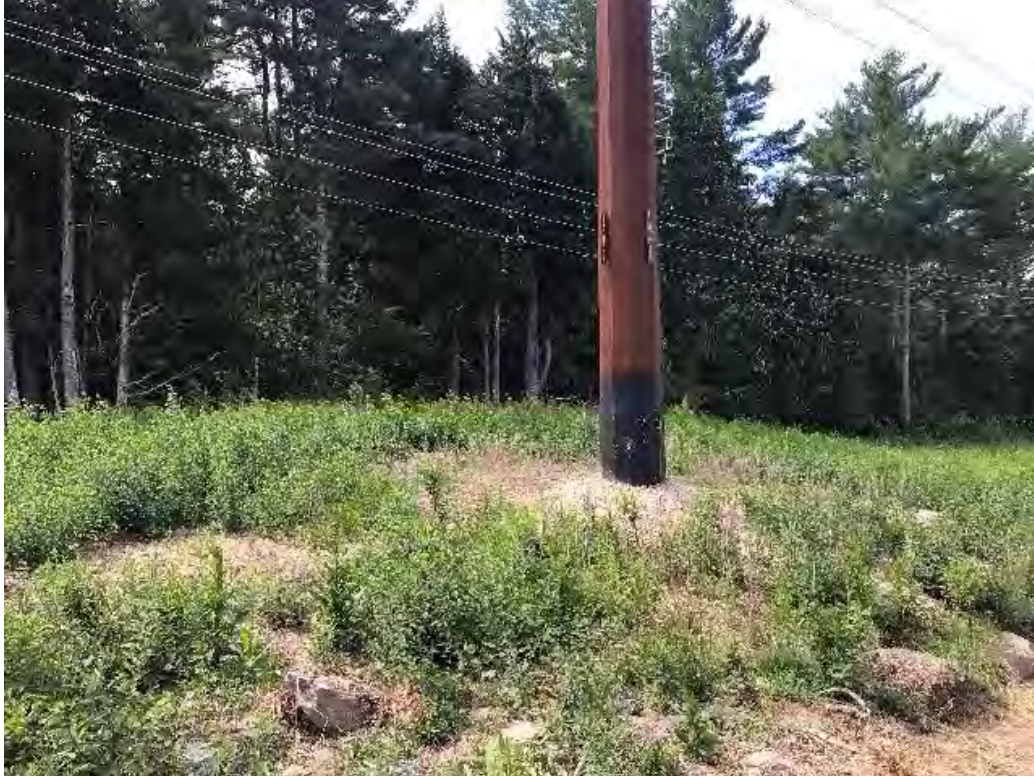
Fig 5: Str. 50 work area re-vegetating. Viewing south. (08-03-20).
