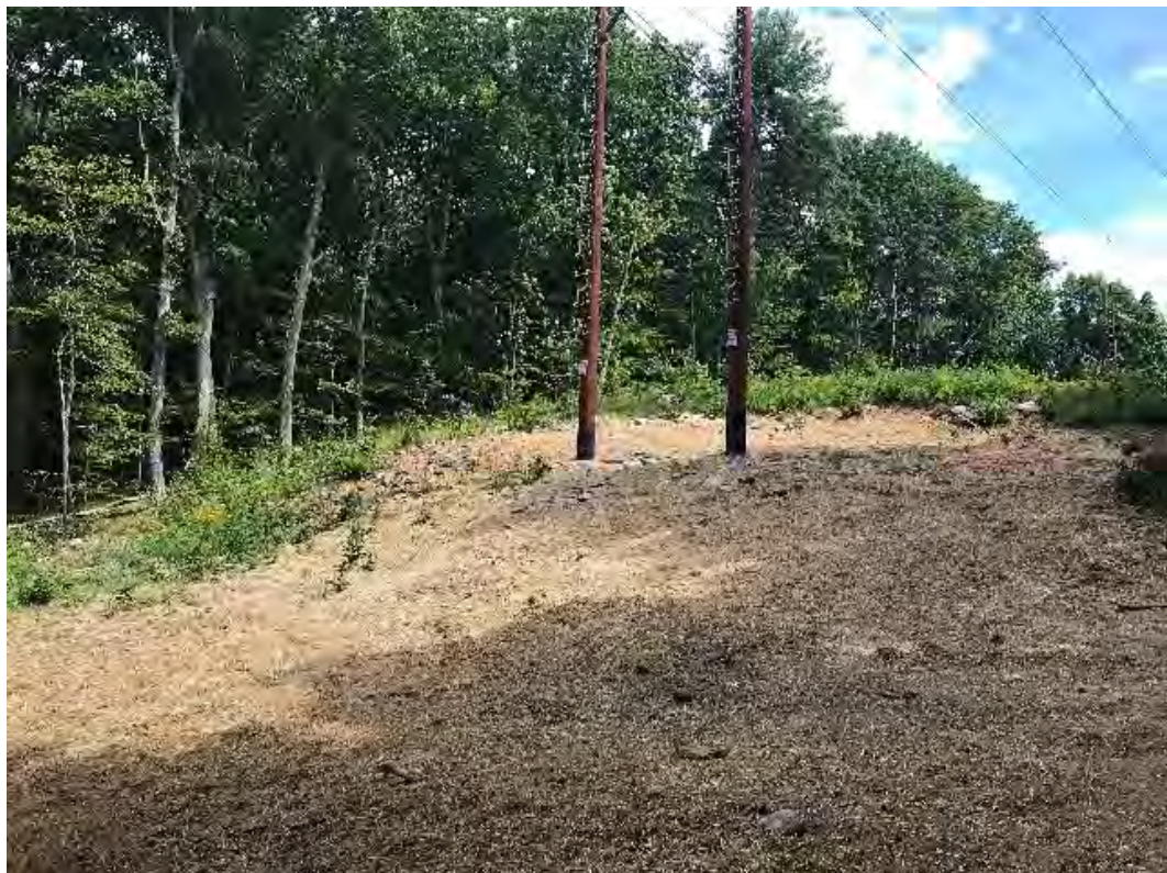
Fig 8: Str. 57 work area mulched and seeded. Viewing northeast. (08-03-20).
