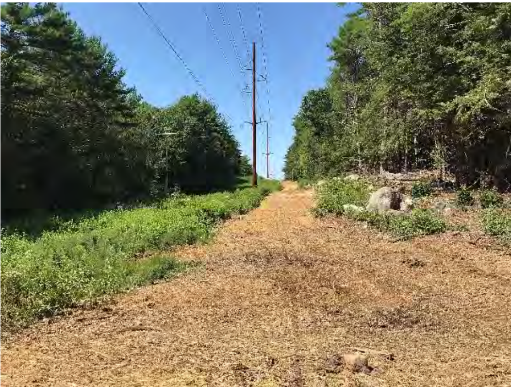
Fig 12: Access road from Strs. 54 to 53 seeded and mulched. (08-05-20).
